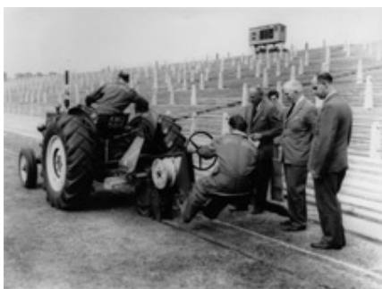
Murrayfield, Summer 1959. Laying the electric blanket during the summer of 1959. Second from the right is D.S. Kerr, Convenor of the Field Committee and, on his right, T. S. Sellars, Head Groundsman.
