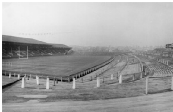
Murrayfield, post-1936. The photograph shows the North and East terracings, complete with score box, and the original West Stand with the North Wing stand which was added in 1936.
